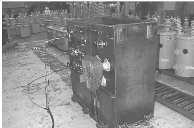
Fig. 1. Test transformer under load test.
